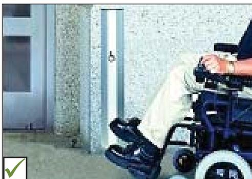
*Touch activation device can accommodate a wider range of users (e.g., can be operated by foot or foot rest).*
