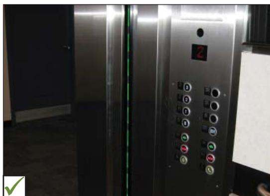
*Elevator sensor door and floor registration buttons.*
