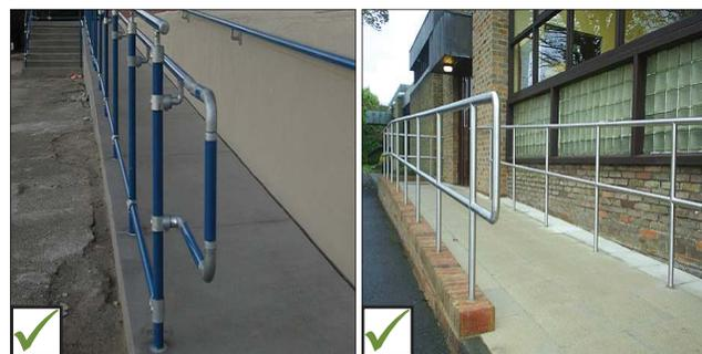
*Ensure handrail extensions do not obstruct path of travel or create hazards.*
